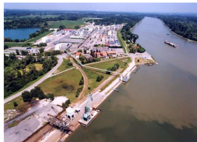
Lauterbourg : usine DOW FRANCE (chemistry)
